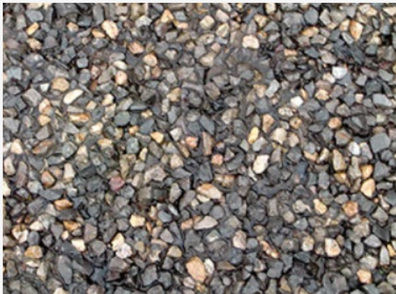
Colored stone in existing asphalt
